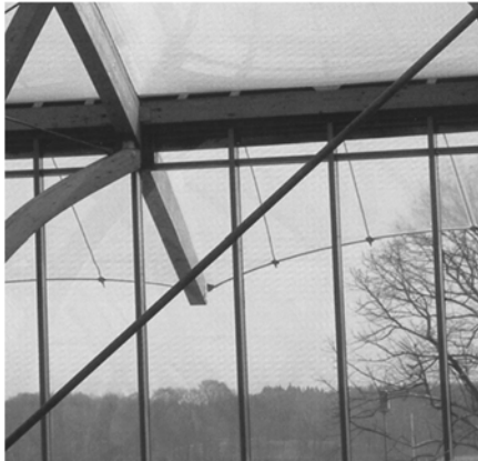
Figure 3: Warm bath Prienavera , ETFE foil cushion as roof covering and transparent canopy (mechanically prestressed single-layer ETFE foil), photo K. Moritz 2001
