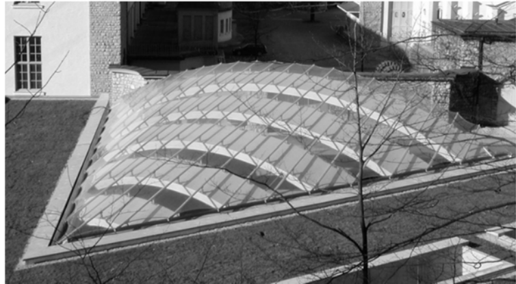
Figure 4: Infocenter Walchensee power plant in Kochel (mechanically prestressed single-layer ETFE film), photo K. Moritz 2001
