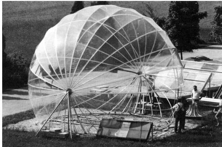
Figure 2: Sphere - Temporary ETFE foil construction at the International Solar Forum 1980 in Hamburg [6].
