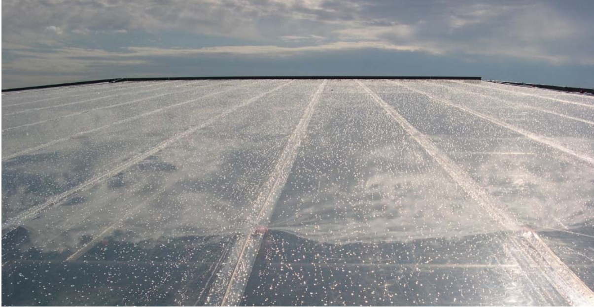
Figure 5: AWD-Arena (today's name HDI Arena) in Hanover, 10,000 m 2 cable-supported ETFE foils, single-layer, mechanically prestressed, Photo K. Moritz, 2004
