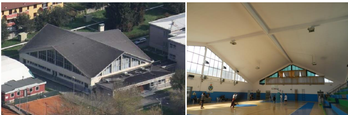
Figure 1. The Codogno sport hall: aerial view (left) and the interior (right).
