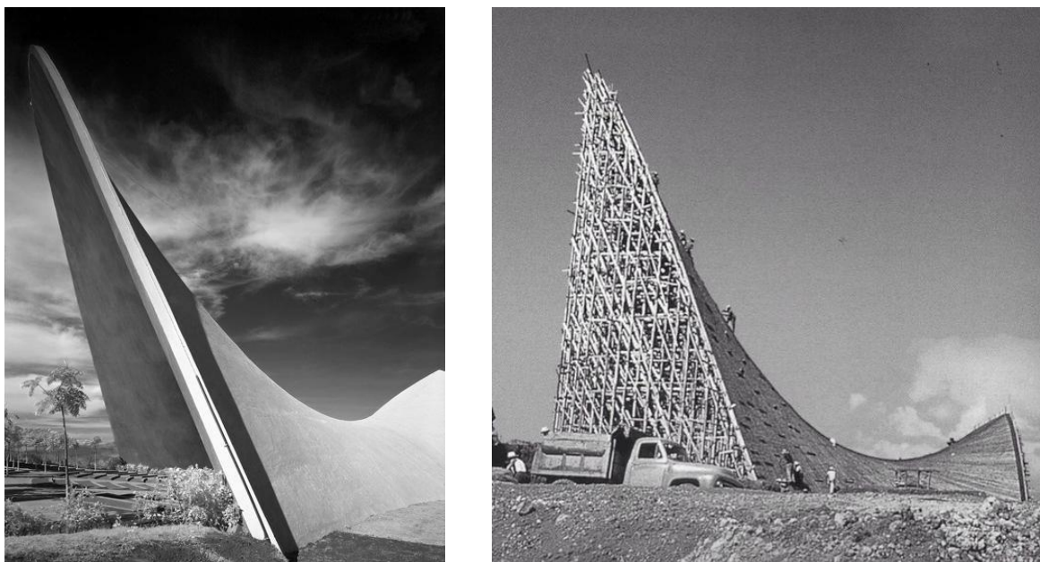
Figure 3. The Cuernavaca chapel finished and under construction.
