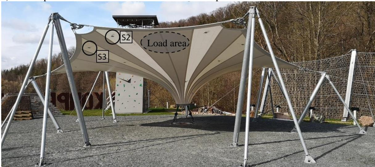
Figure 11: Built demonstrator; location of the considered sensors and load area
