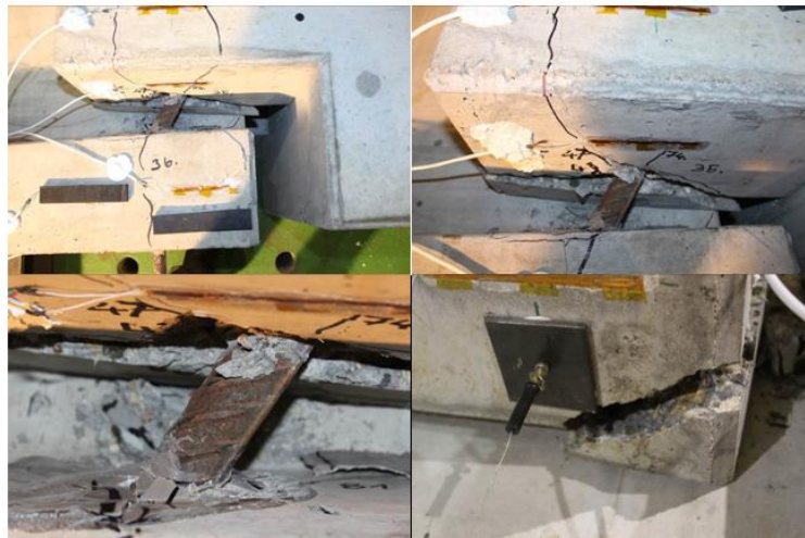
Figure 14: Specimens #3 – Failure by dowel yielding and concrete spalling
