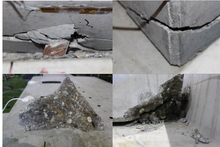
Figure 12: Specimens #2 – Failure by dowel yielding and concrete spalling
