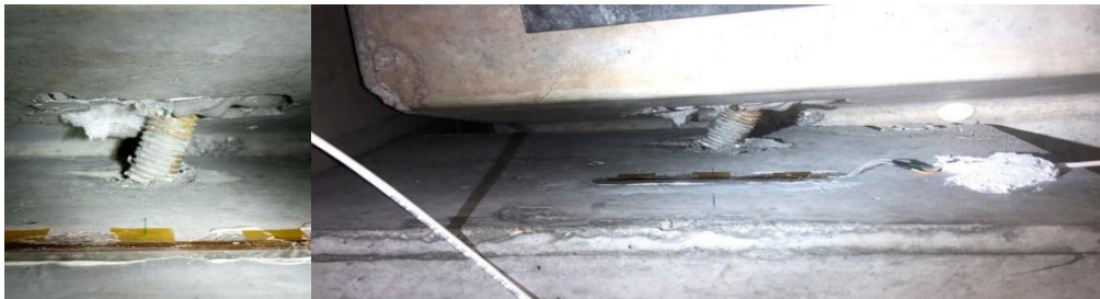
Figure 10: Specimens #1 – Failure by dowel yielding
