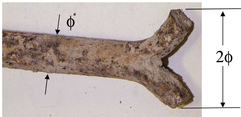
Figure 6: Fish-tailed anchorage of bending reinforcement. From a residential building in Genoa, Villa Grüber park, Genoa, Porcheddu Building Company , in-between 1920-to-1930. main geometric ratios.
