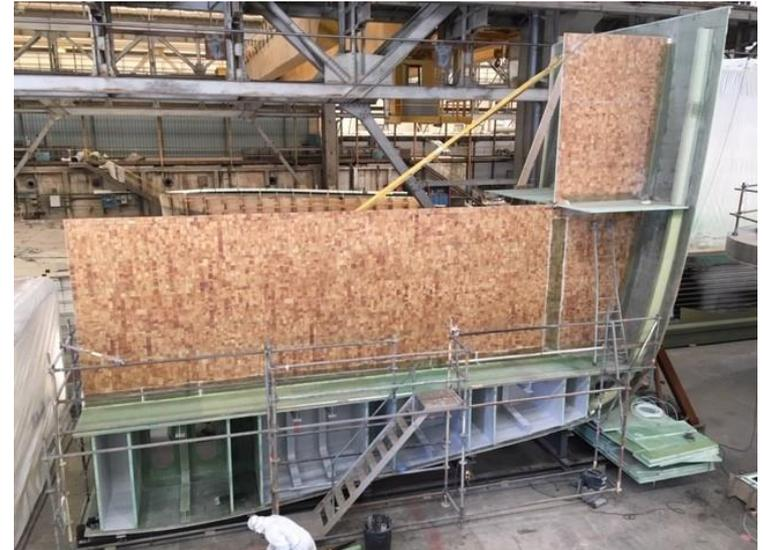
*Demonstrator currently under construction at iXblue showing **laminated** and **sandwich** construction*
