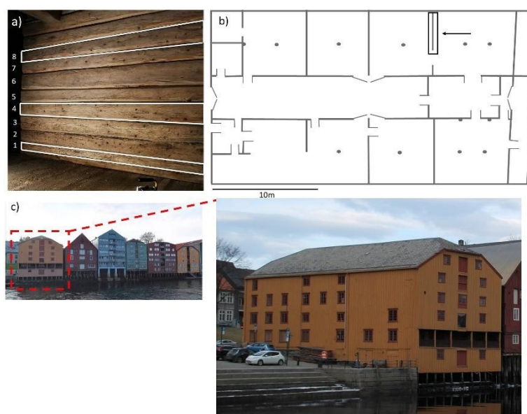
Figure 1: a) Selected logs; b) Plan of the ground floor. The studied wall is circled, and the arrow indicates the tested side; c) The warehouse studied in Trondheim.
